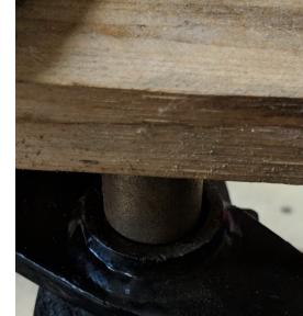
Inserting the new bushing with a piece of wood
